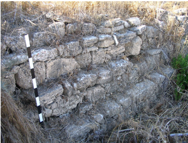
Fig. 3 – Check dam (R. Scott Moore).
