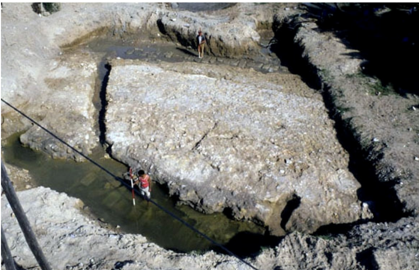
Fig. 8 – South mole near Roman harbour entrance, looking SSE. The figure in the foreground stands on the facing of (submerged) cut stone blocks inwards towards the harbour and the background figure stands on the facing southwards to the open sea. (Photograph by author).
