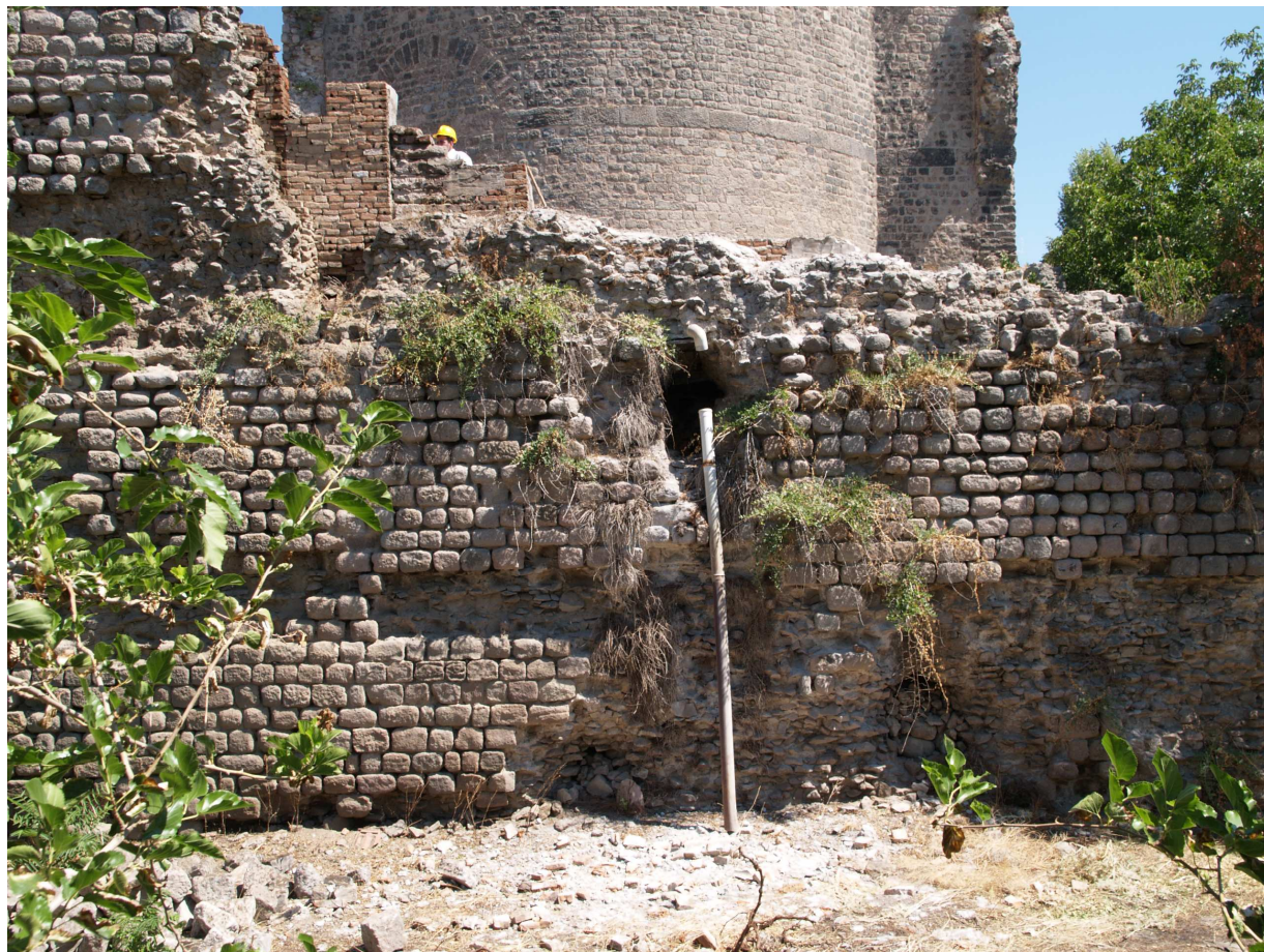
Fig. 16 – Retaining wall of the Red Hall in Pergamon (BACHMANN 2006).
