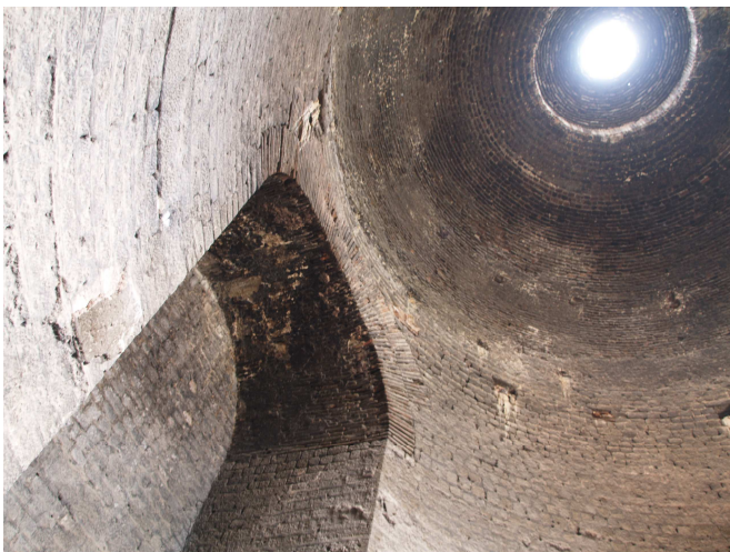
Fig. 15 – Dome of the southern tower of the Red Hall in Pergamon (BACHMANN 2006).
