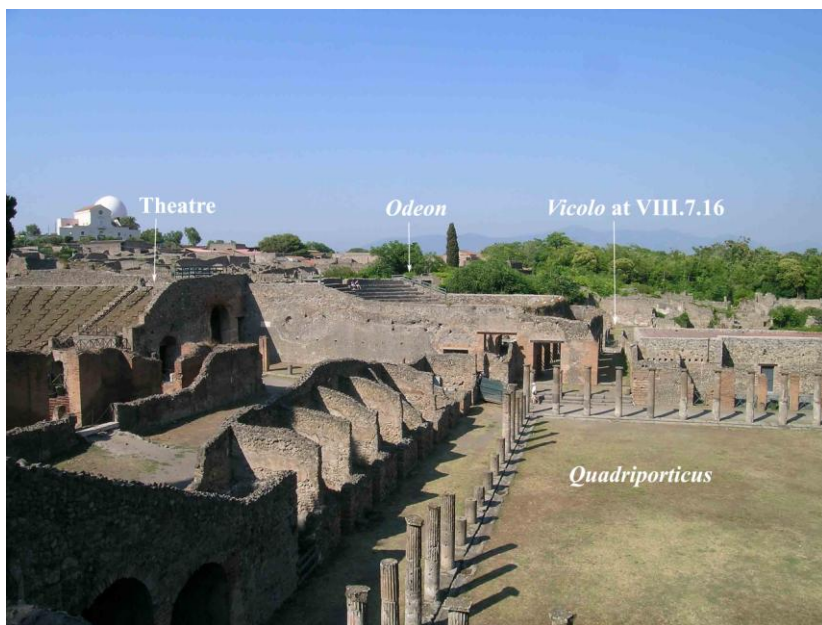
Fig. 33. The Quadriporticus with its entrance from the vicolo of VIII.7.16, looking east.
