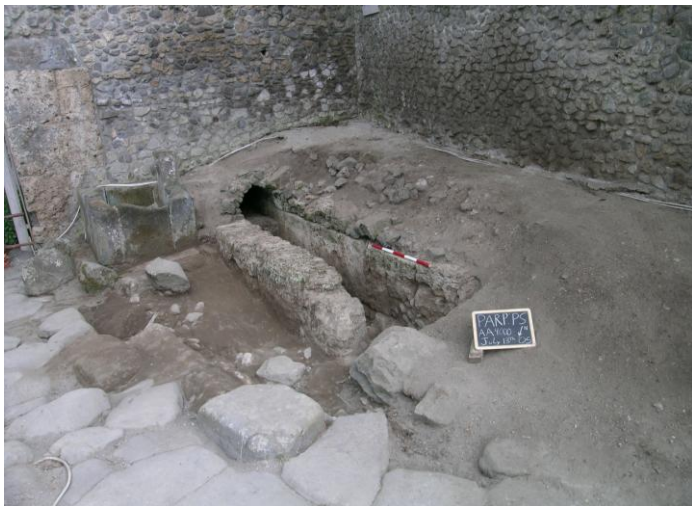
Fig. 25. The city drain at the southern extent of the via Stabiana , passing behind the Porta Stabia fountain and through the gate itself.
