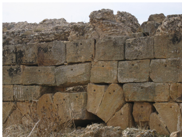
Fig. 8 - Cavea Wall Section – Upper Section in Opus Caementicium .
