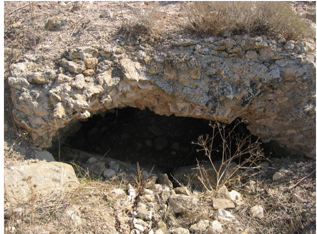
Fig. 11 - Rear Cavea – Stone Archway Opening.
