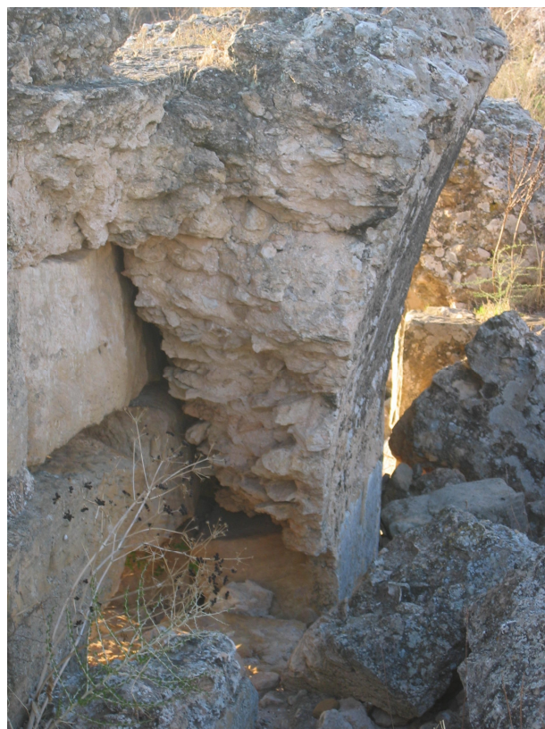
Fig. 9 - Cavea Wall Section – Rear Segment.
