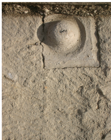
Fig. 10 - Detail of the pivot stone of the western gate probably erected in 174 BC, ten years after the foundation of the Roman colony.
