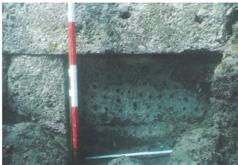
Fig. 8. Detail of the opening with a lead grid (P), in the NW corner of vat 1.
