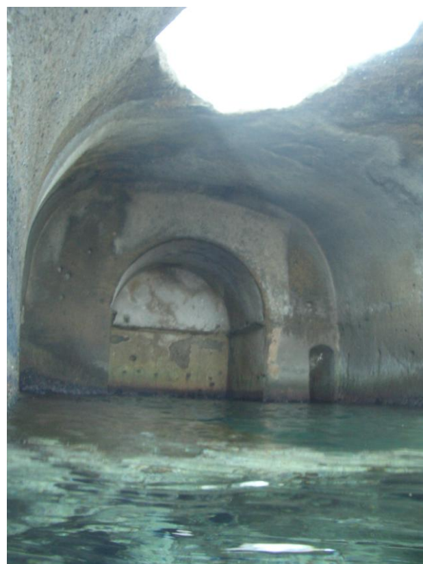
Fig. 17. View of the quadrangular apse and of the tunnel (O) of vat 3.
